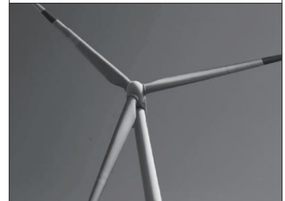
wind blade deformation inspection
