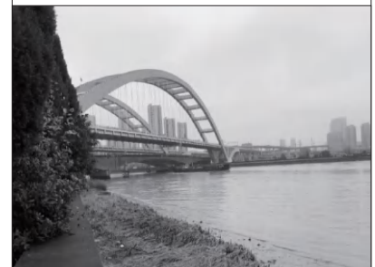
deformation monitoring of bridges and tunnels
